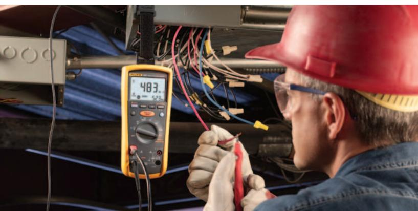
Avoid electrical shorts by testing the insulation resistance on cabling.
