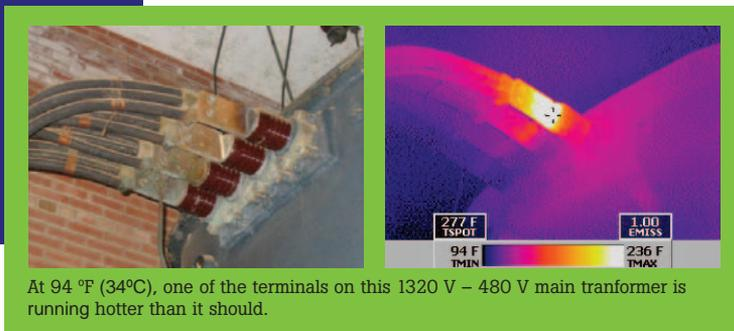
At 94 °F (34°C), one of the terminals on this 1320 V – 480 V main transformer is running hotter than it should.
