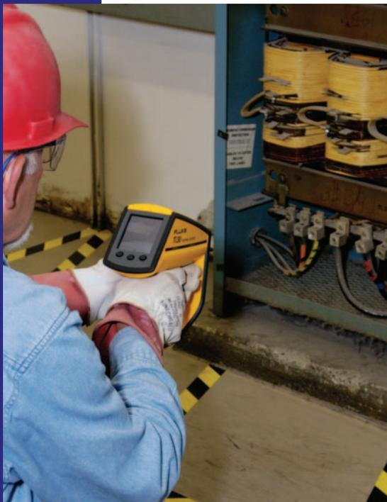
Power and distribution transformers change electric current from one voltage to another. They accomplish this process when electricity flowing through a coil at one voltage induces current in a second coil. The amount of change is a function of the number of windings on the coils.
