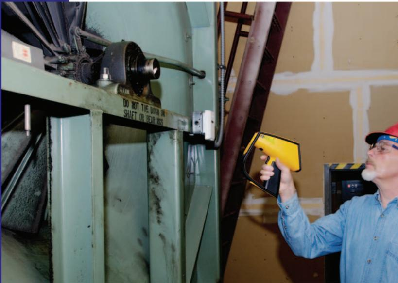
Many facilities monitor this type of equipment on a regular basis, because often a simple problem like lubrication can be spotted and fixed inexpensively, before the entire unit burns out. Such strategies fall under the general heading of predictive maintenance (PdM).
