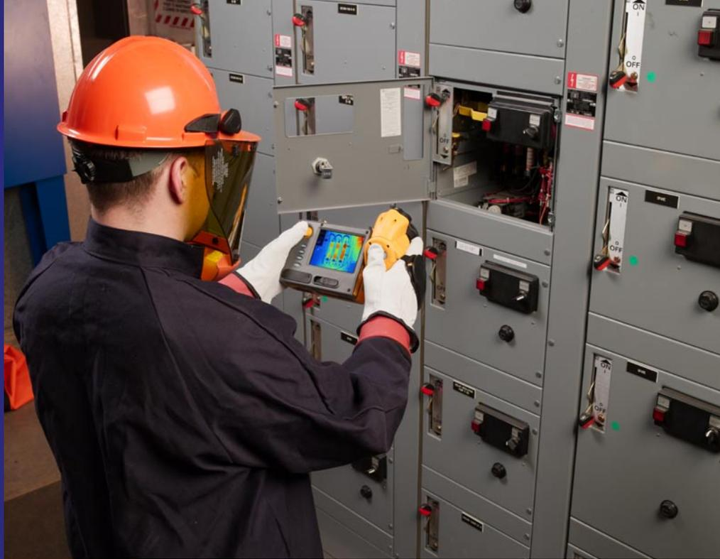
like bus bars and any large metal electrical connectors, you need to adjust the emissivity value on the imager.
