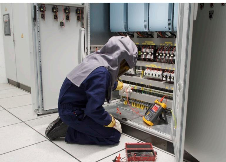
Rob Withey uses a Fluke ScopeMeter to check the output voltage that drives Peak 2 Peak conveyor motors.
