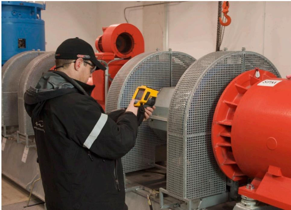
Rob Withey uses a Fluke thermal imager to check temperature on bearings and gearbox housings on the 335 kW (450 hp) motors in the Peak 2 Peak main drive room.
