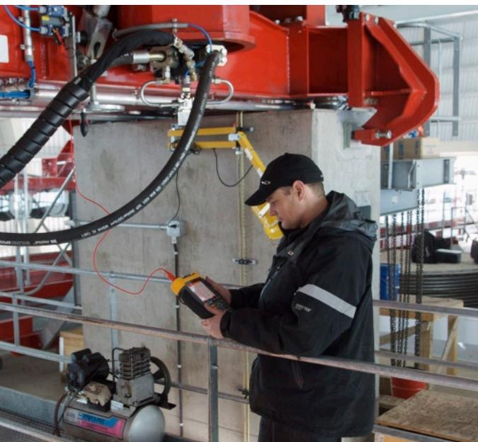
The Whistler/Blackcomb Peak 2 Peak gondola has many safety and redundant electrical systems. Rob Withey uses a Fluke ScopeMeter to look for voltage drop at a switch.
